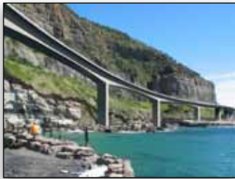
Lawrence Hargrave Bridge, AECOM Maunsell Australia.
