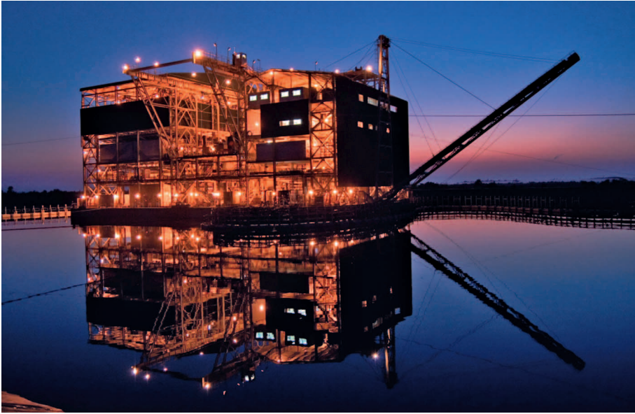
The floating wet plant at the QMM ilmenite project
