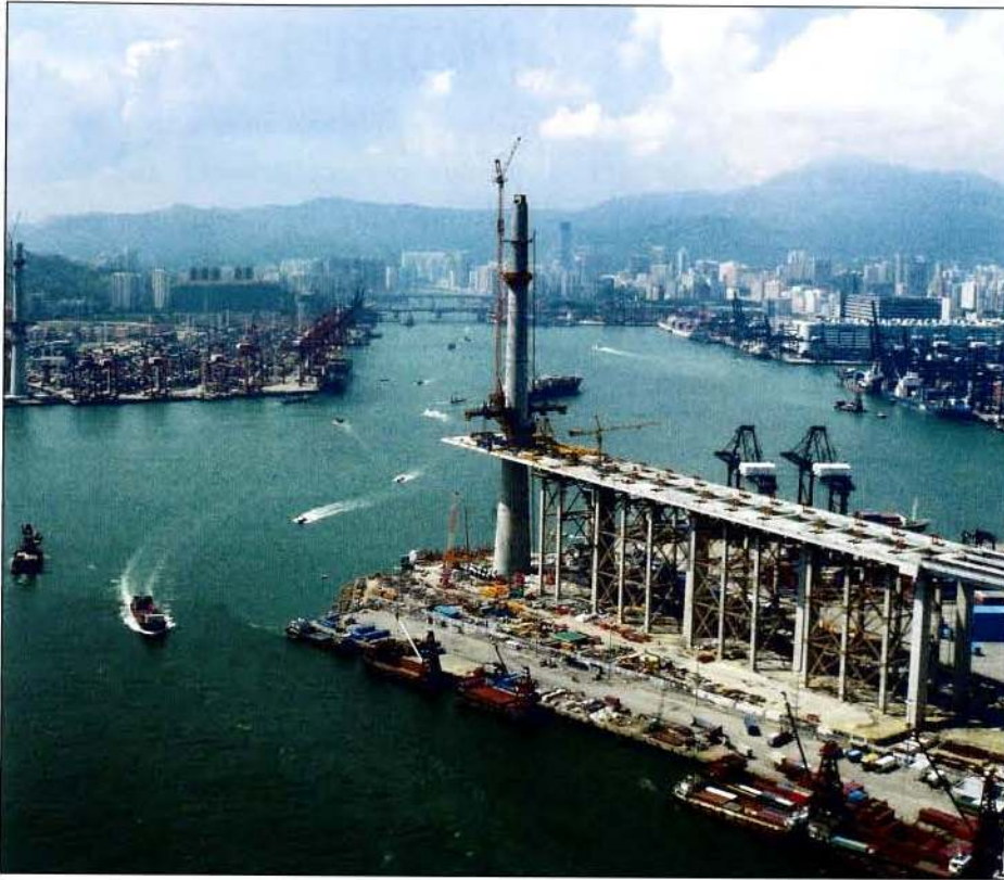
Fig. 3: Stonecutters Bridge Under Construction
