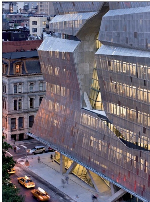
New York's 41 Cooper Square project by Morphosis architects.
