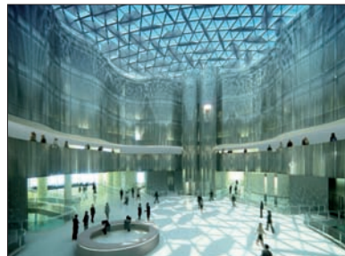
Craig Schwitter of Buro Happold reviewed a series of projects in collaboration with Chuck Hoberman. This atrium's internal facades are shaded but the atrium floor receives dappled sunlight adding an aesthetic dimension to the shading solution.
