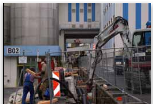
KELAG Wärme laying new district heating infrastructure documented in Bentley sisNET.
