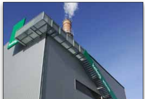
A KELAG Wärme district heating plant in Austria generates hot water for district heating services.
