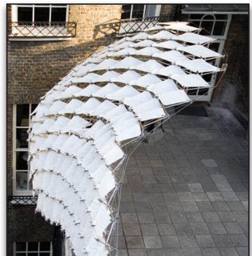
These membranes contribute considerably to the stiffness of the overall structure
