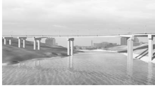
Bridge after applying fog.
