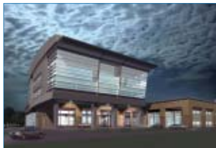
▲ "Visualizing something two years before it's built helps with decision making and enables us to explicitly communicate with our clients," NBBJ's Drew Burgess said.
