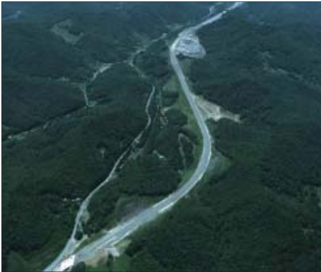
One of the largest projects in NCDOT's history, I-26 opens to traffic summer 2003.
